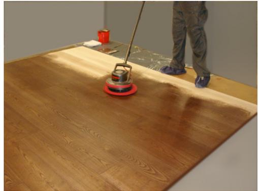
**Note:** Some wood species, like Douglas Fir, will naturally absorb more oil. Pre-finishing treatments can make the wood grain very open and dry, causing more absorption. While doing (D) above, check for dry spots or an uneven appearance. **Only if necessary**, squeeze **small** amounts of oil onto the spots and spread with the buffer. When the appearance of the section is consistent, buff the entire area one last time and continue the application.
